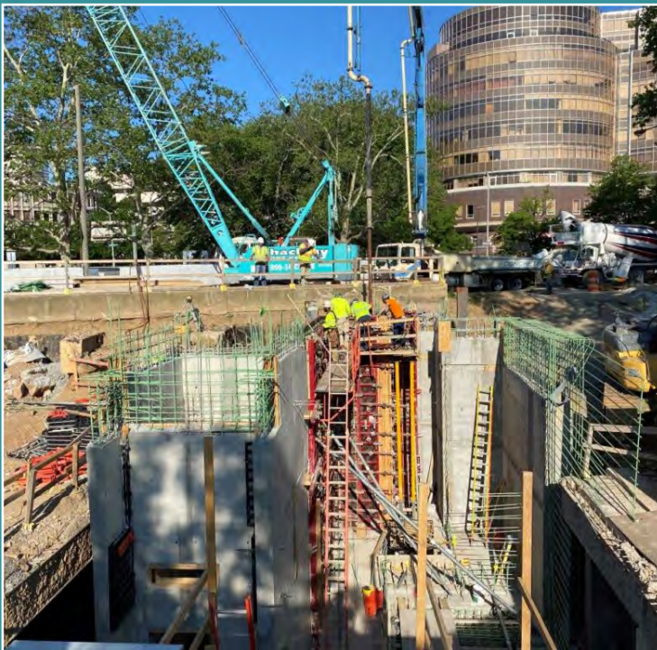
The south entrance staircase walls have now been constructed.
