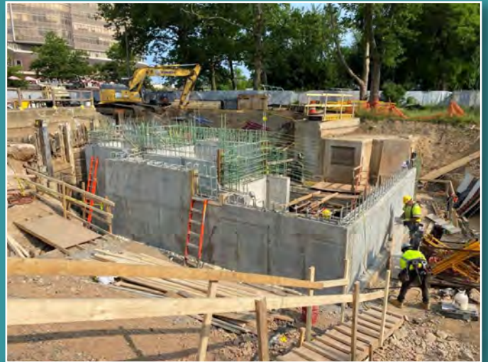
The entrance staircase roof walls have been partially constructed.
