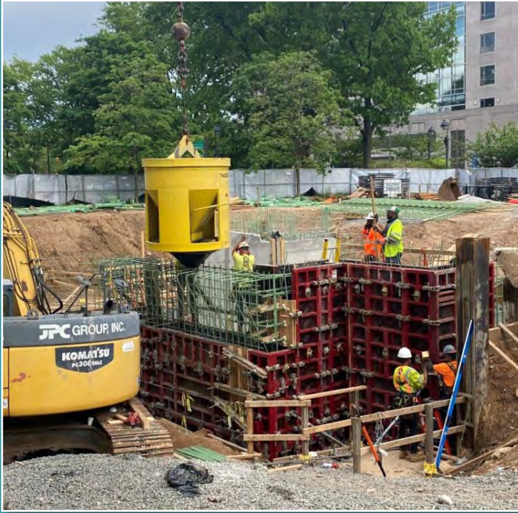
The north entrance staircase walls have now been constructed.
