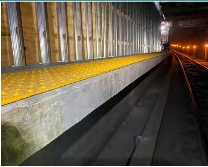
Tactile warning surface has been installed along the Track 1 platform edge.
