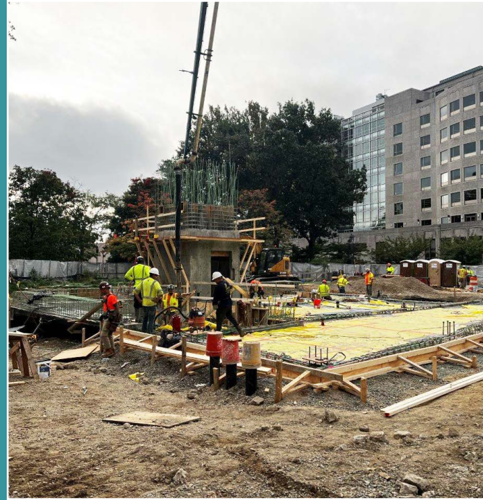
Final backfilling has been completed under the headhouse floor slab.
